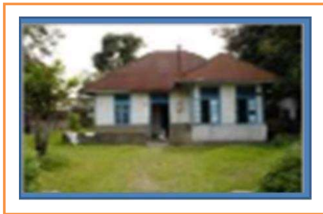
Figure 6. Ex Customs Building for Medan Labuhan
