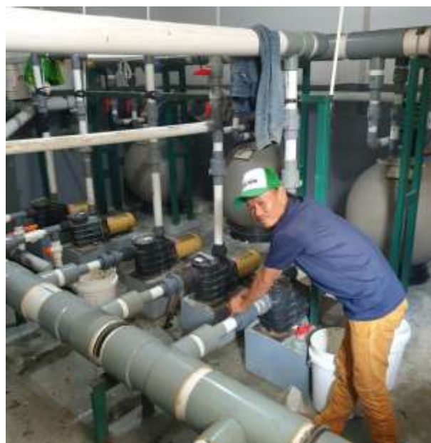
Figure 1. Repairing the condition of Water Circulation Machine
