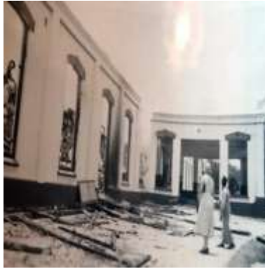
Figure 2. The Siantar Hotel Building which was Burnt by Youths Source: https://theindoproject.org/a-festive-massacre/
