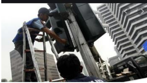
Figure.2 Traffic Lights Broken
