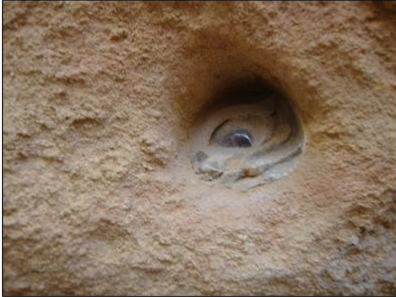
Figure 8. Loss in the Stone as a Result of the Presence of One of the Fossils within the Formation of the Stone
