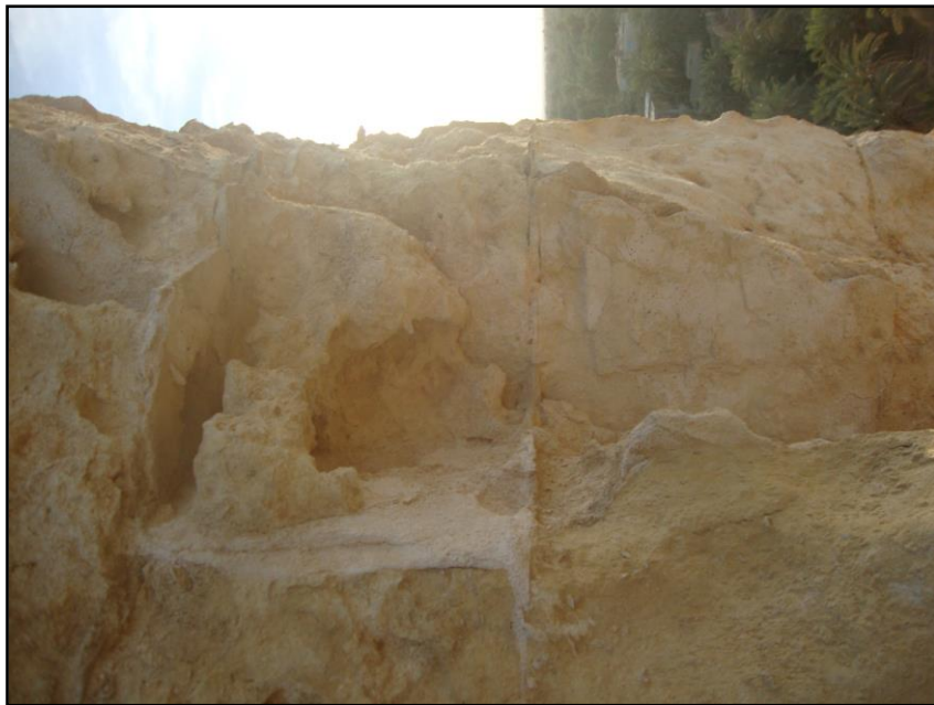
Figure 5. The Erosion of Stone Layers in One of the Temple Walls
