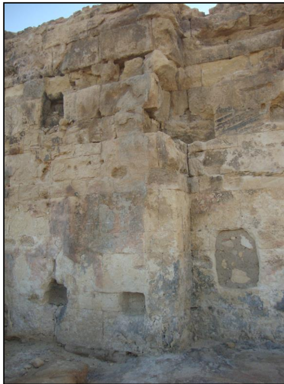
Figure 7. Erosion in the Stones of One of the Facades of the Temple as a Result of Wind Erosion
