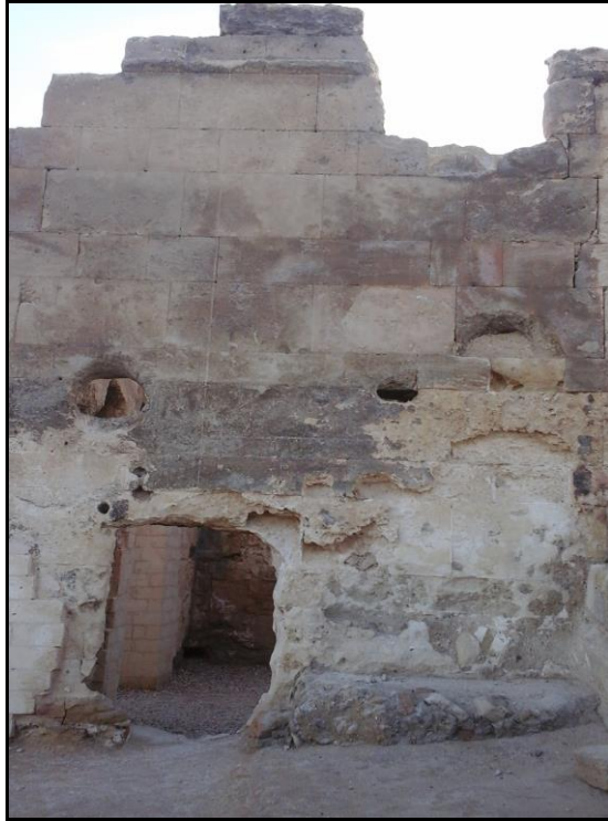
Figure 4. The Erosion of Stone Layers as a Result of Salt Dissolution
