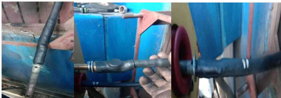
Figure 8. Motor Terminal Cable Repair
