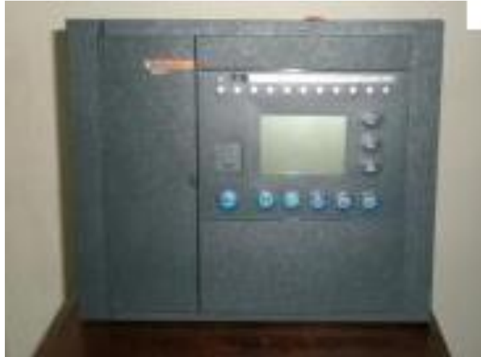
Figure 4. Schneider Protection Relay
