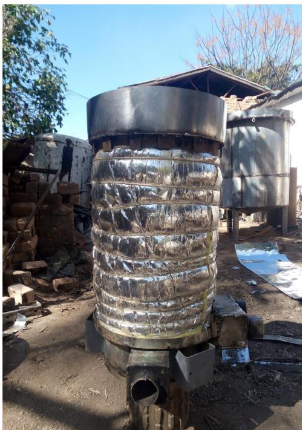
Figure 1: The Tank Wrapped in Rock Wool
