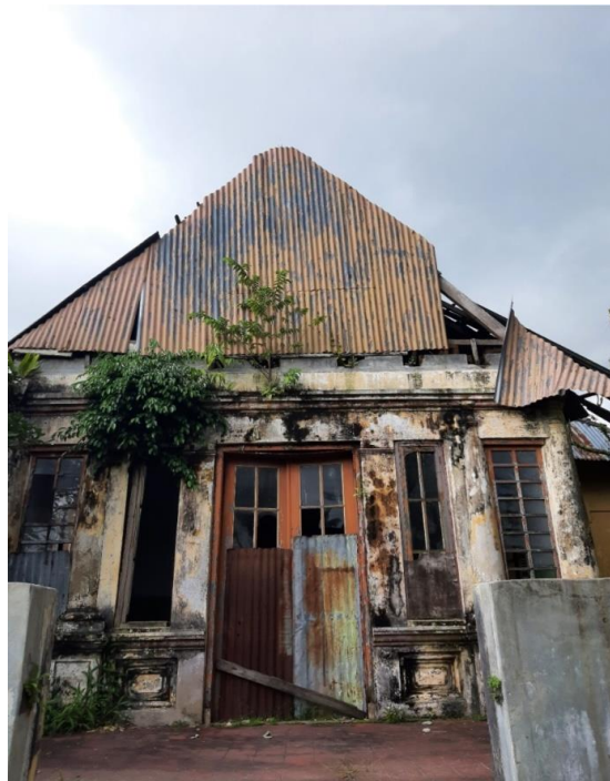
Figure 3. Former Raja Siantar House at present in 2022
